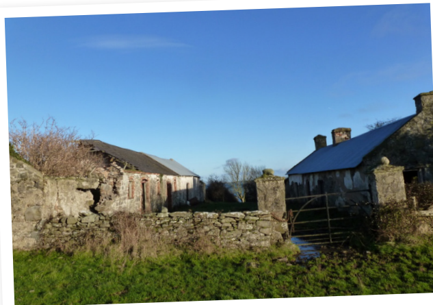
A disused farm building - one of the many sites surveyed for barn owls
