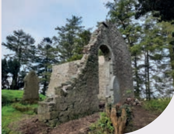
Derryvullan Old Church Ruins Stabilisation and Conservation
